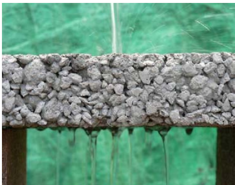
Pervious Pavement Source: Clear Creek Solutions; LID Hydrology and Hydraulics Presentation
