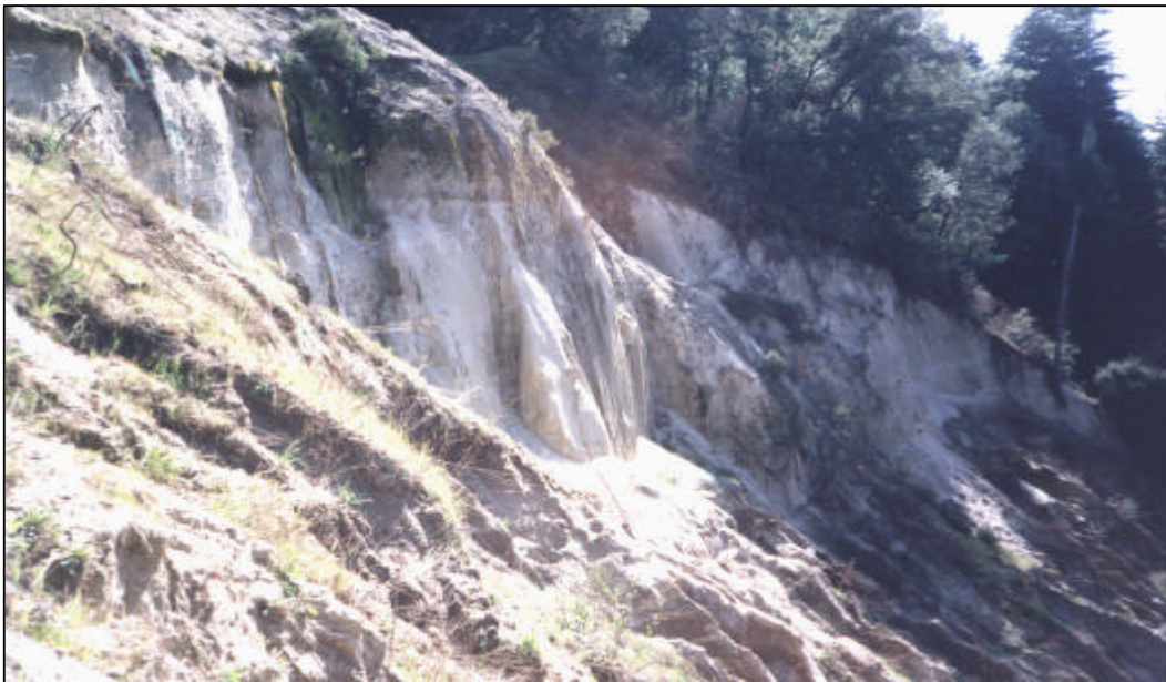
Figure 3.2: Eroding Road Cuts on Bean Creek Road Within Santa Margarita Sandstone
