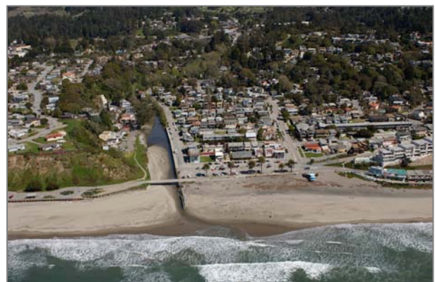
Figure 5-11: Rio Del Mar Esplanade/Flats Source: California Coastal Records Project.
