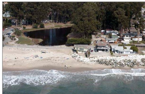
Figure 5-8: Moran Lake Source: California Coastal Records Project, 2012.
