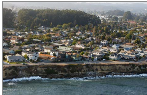
Figure 5-9: East Cliff Drive at Pleasure Point Source: California Coastal Records Project, 2012.
