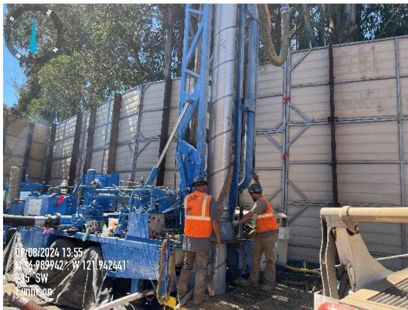
Figure 6: Cunnison Well drilling. Photo courtesy of SqCWD.
