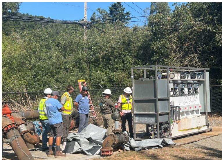
Figure 17: Hexavalent Chromium treatment pilot. Photo courtesy of SqCWD.
