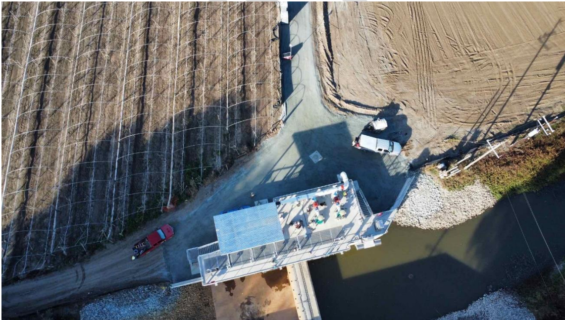
Figure 18: College Lake Project Weir. Photo courtesy of PV Water.
